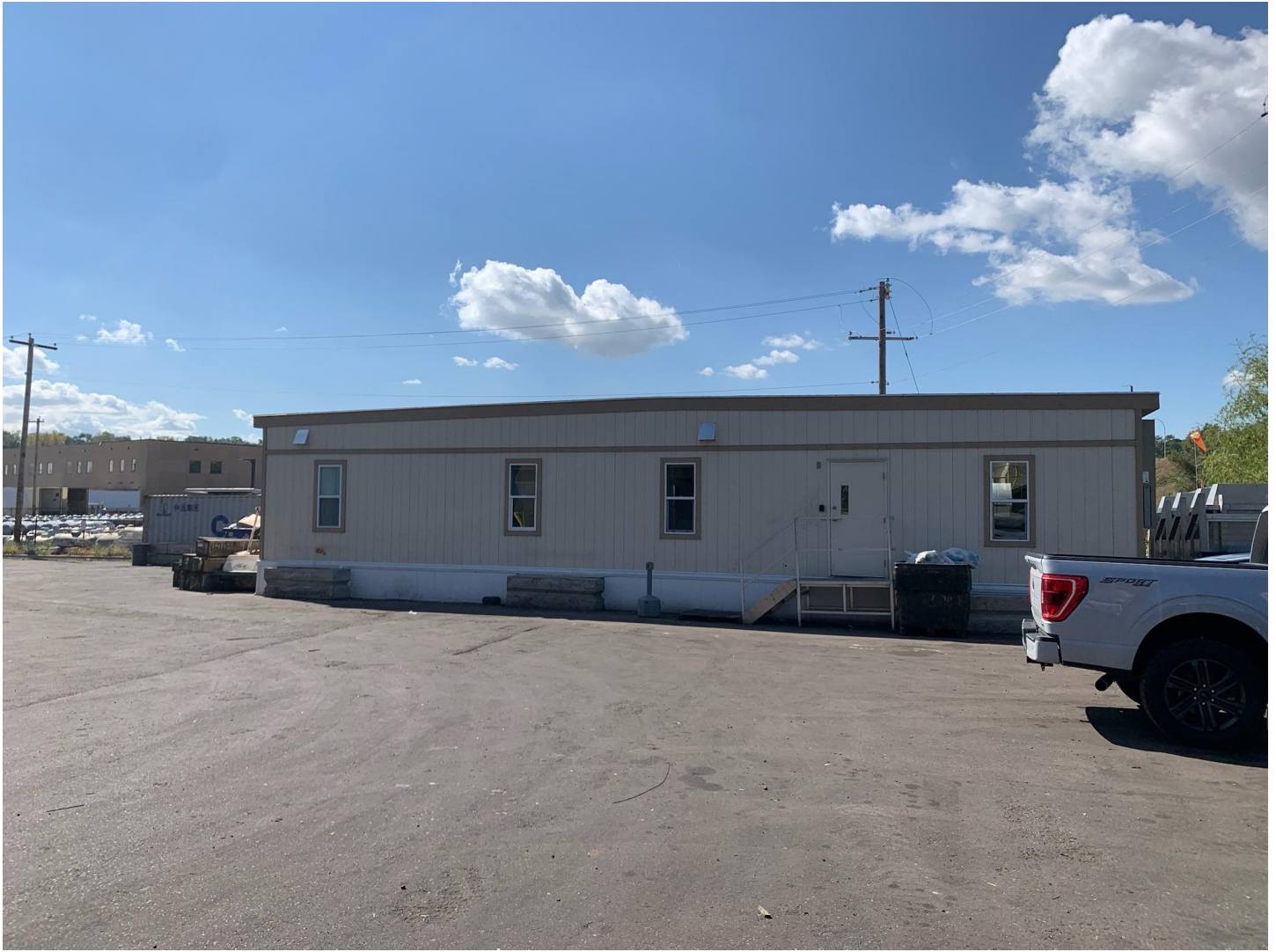
Photograph of Existing Temporary Building at Subject Property (Taken 9/24/2024)
