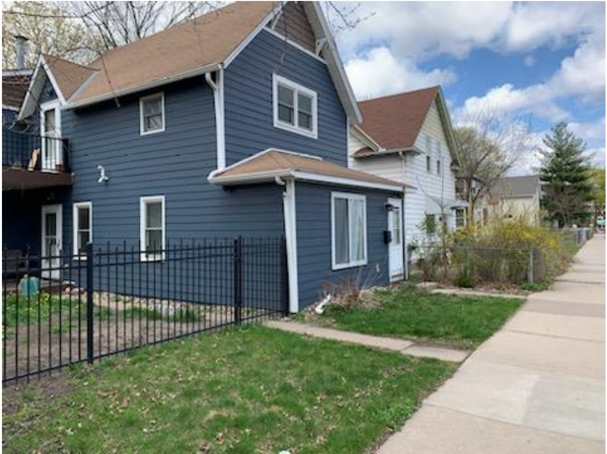
Existing House at 144 2 nd Avenue South Which Has a 10-Foot Deep Front Yard
