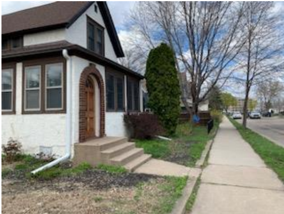
Existing House at 158 2 nd Avenue South Which Has a 10-Foot Deep Front Yard
