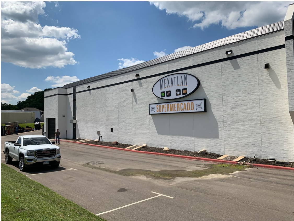
BUILDING FAÇADE FACING CONCORD STREET
