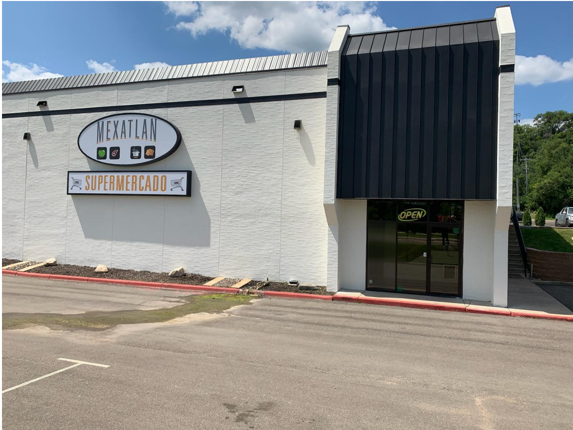
BANQUET HALL ENTRANCE FACING CONCORD STREET
